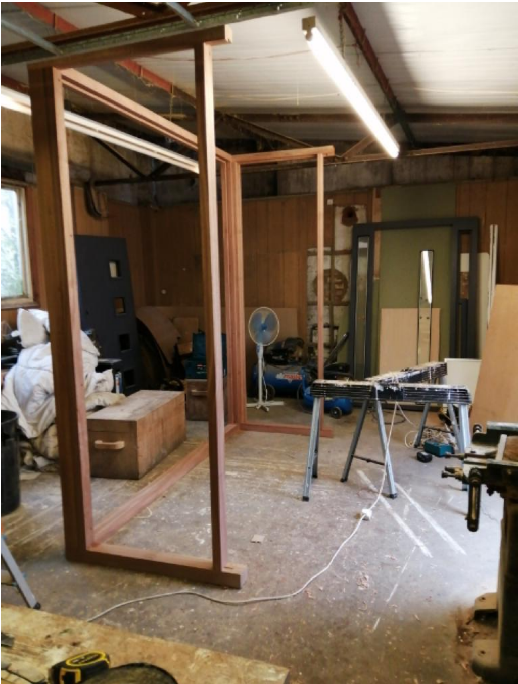
Fig 1 Porch under construction
